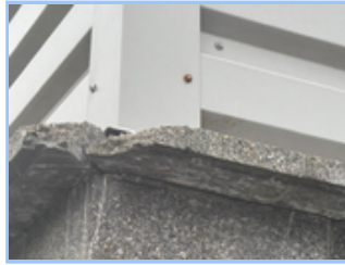
South and East Side of the Station
