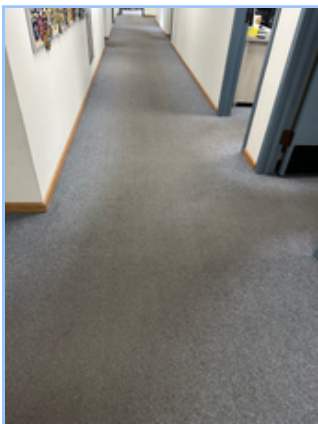
Hallway outside locker room.jpg
